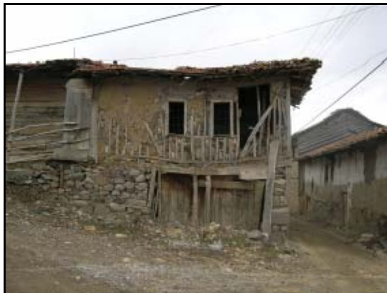
Figure 4.11 Composite structure: Stone masonry first floor and timber-frame with stone infill (Ortabayındır Village).
