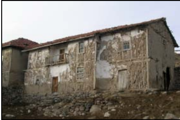
Figure 4.9 Timber-framed structure with sun-dried brick infill (Yuva Village).
