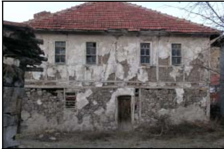
Figure 4.10 Composite structure: Stone masonry first floor and timber-frame with sun-dried brick infill (Yuva Village).
