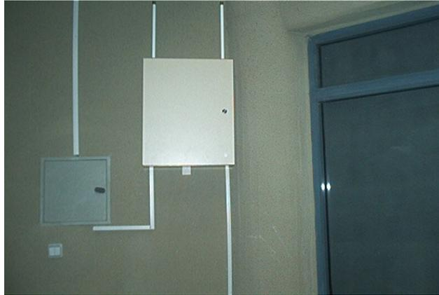
**Figure 9 – Wood Enclosure for WLAN Equipment**
