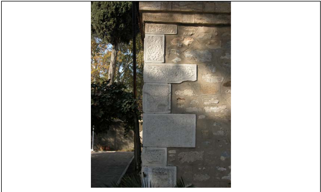
Fig.2.50: The reused stones in Selçuk station
