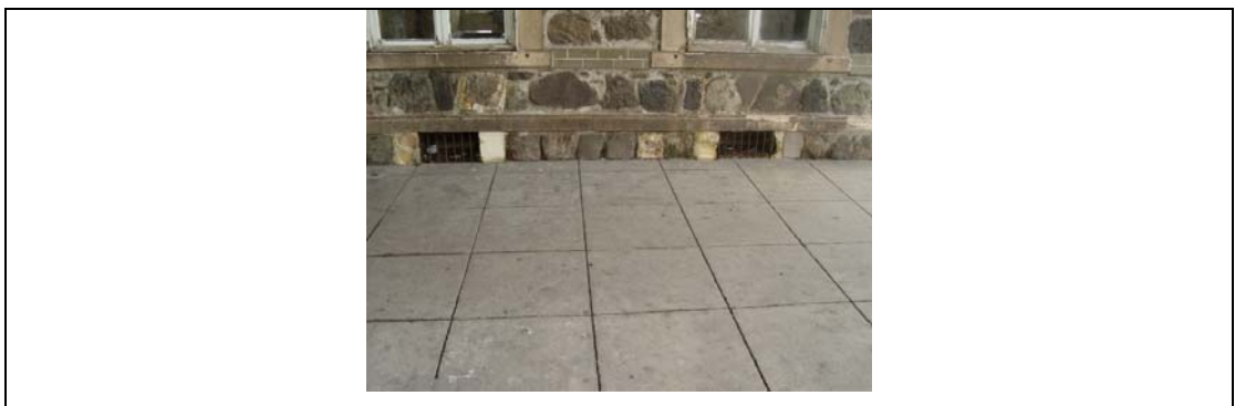
Fig. 2.45: The openings to ventilate the foundation and platform pavement, Kemer station
