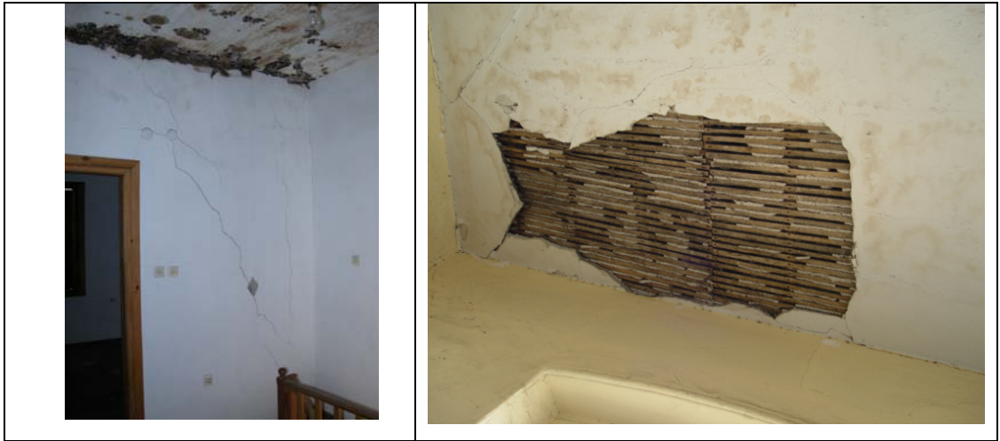
Fig.2.67: Finishing problems in amlık and Kemer main station buildings
