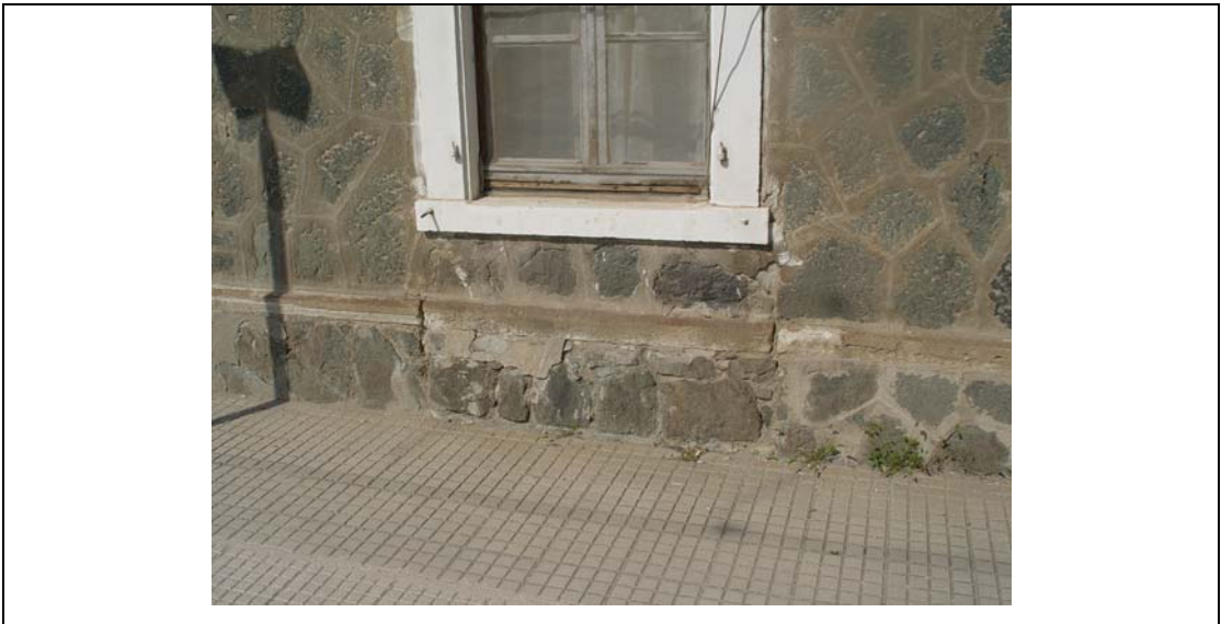
Fig.2.64: Discoloration and cracks in the main station building of Gaziemir station
