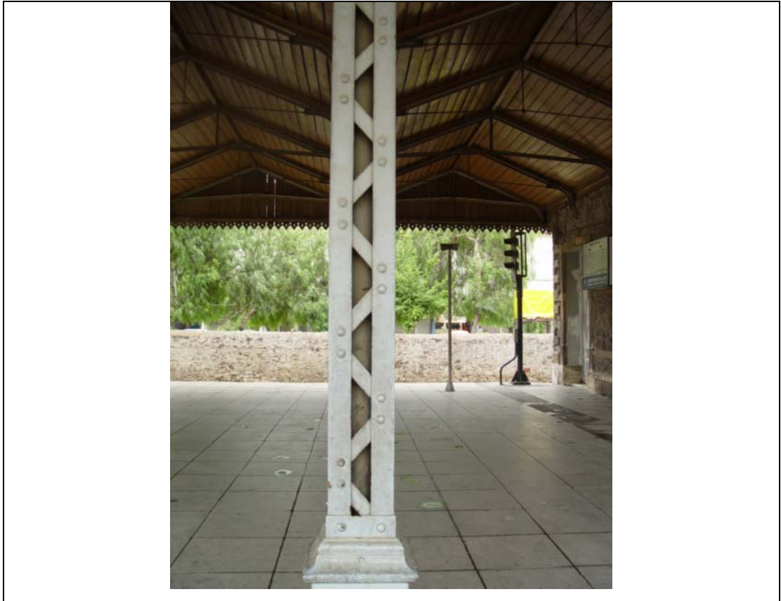
Fig.2.55: Kemer Station shed columns, with water drainage pipe in the middle
