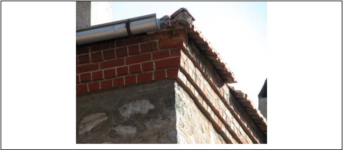
Fig.2.61: The roof cornice of Selçuk main station building
