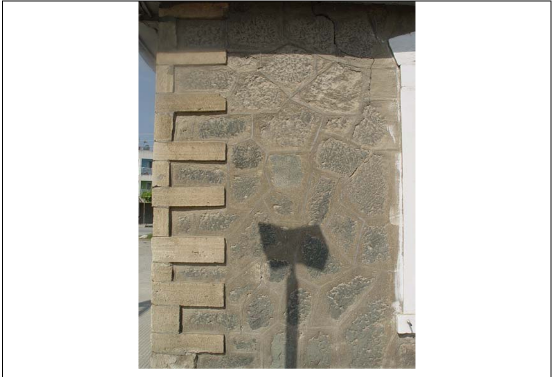
Fig.2.49: Cut stone at the corners, Gaziemir station
