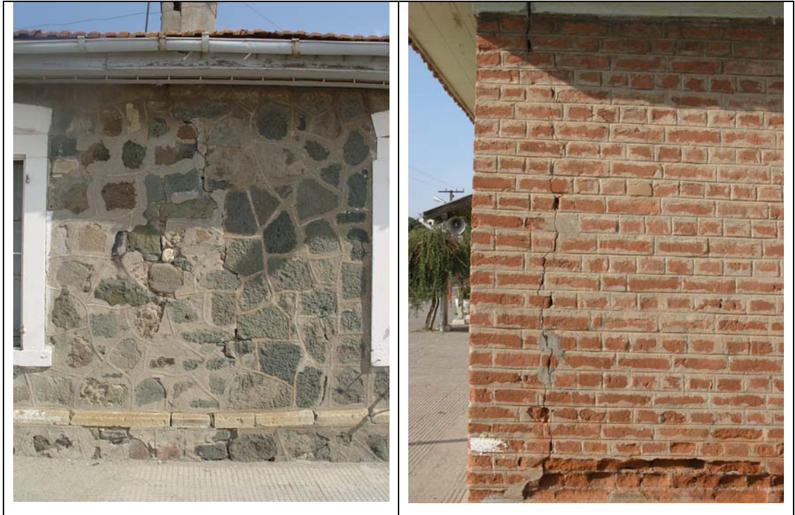
Fig. 2.66: Structural cracks in Gaziemir and Torbalı main station buildings
