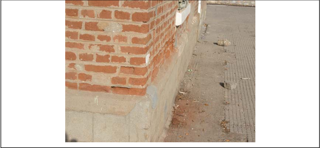
Fig.2.65: Material loss due to rising damp in Torbalı main station building
