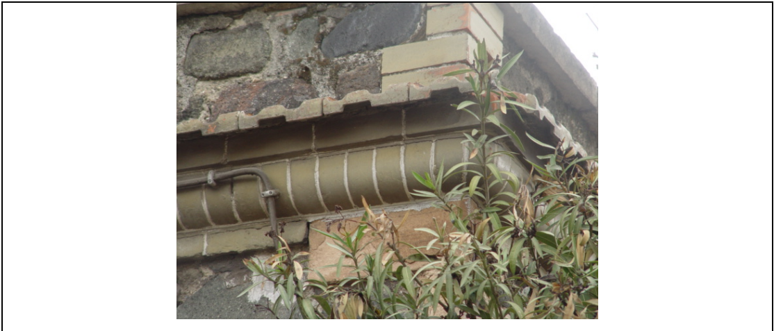
Fig.2.63: The roof cornice of Kemer main station building
