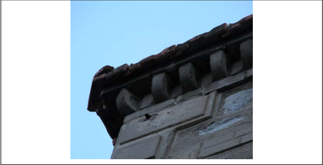
Fig.2.62: The roof cornice of İncirliova main station building
