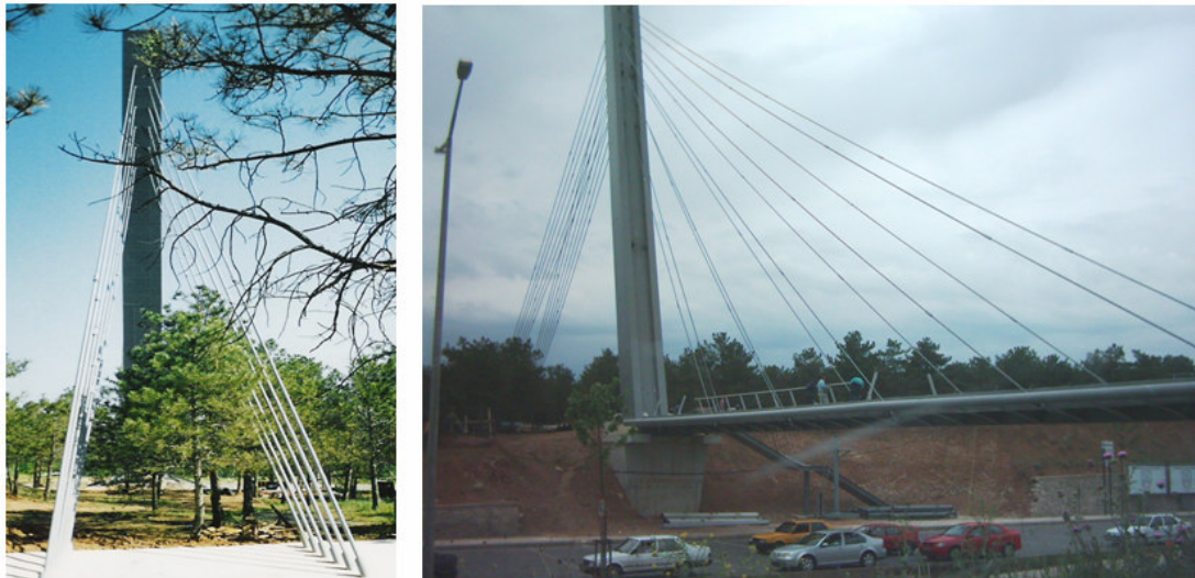
Figure 3-11: Arrangement of the Investigated bridge stay cables
