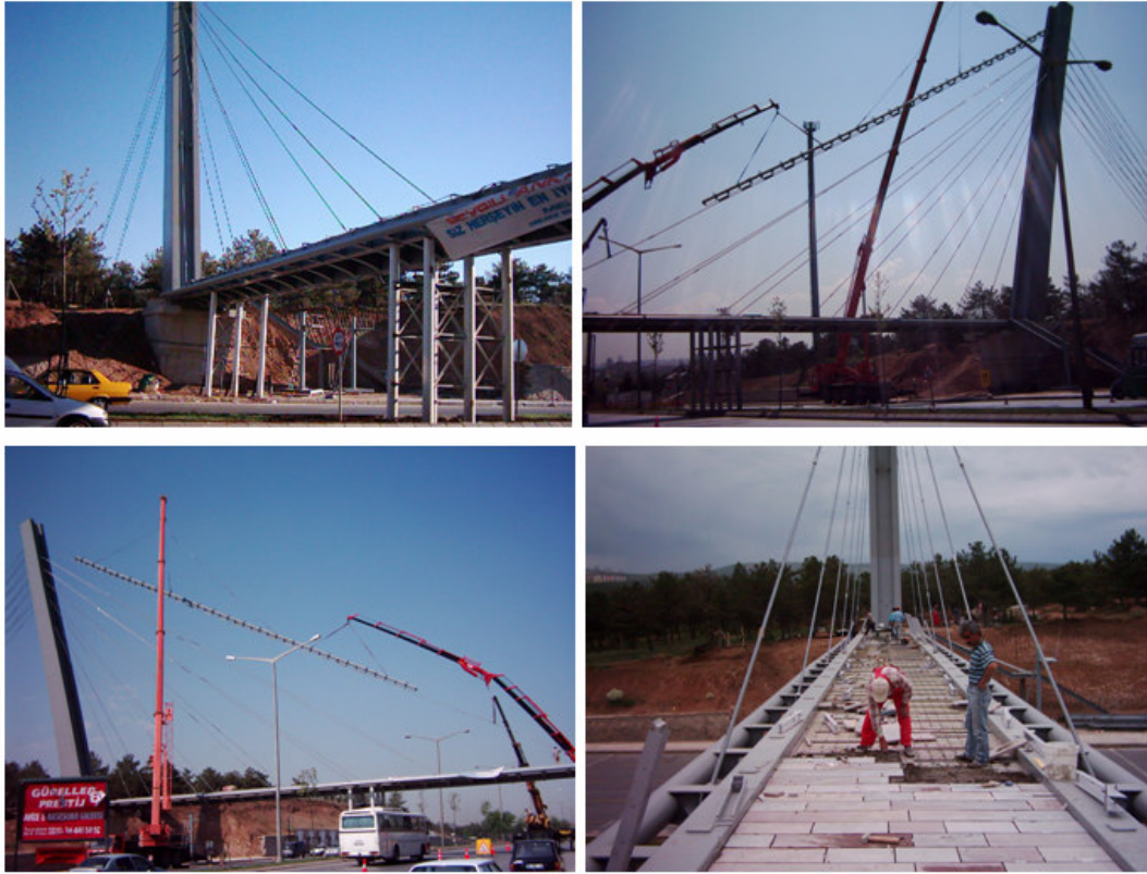
Figure 3-22: Cabling, support removal and tile placement process
