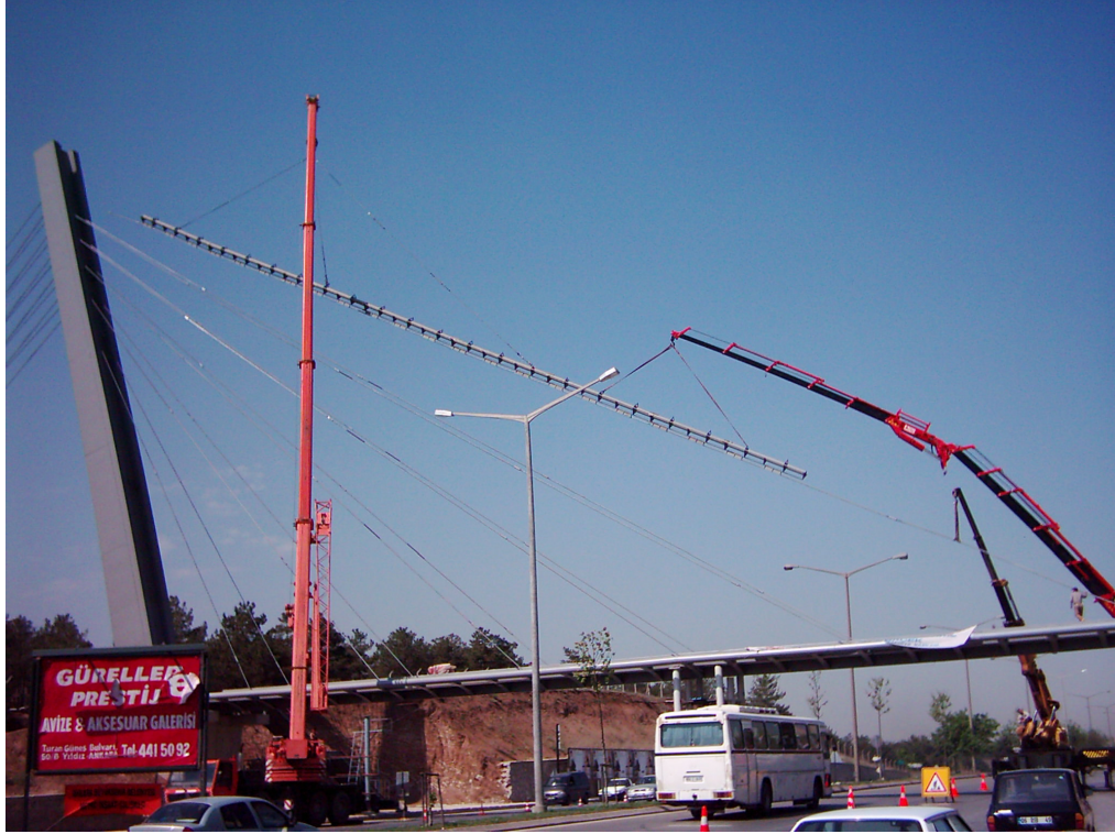
Figure 3-9: The process of connection of the cables and anchoring of structural parts.
