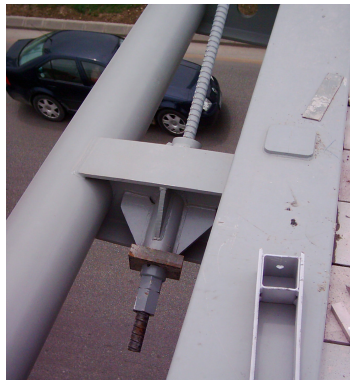
Figure 3-7: The cable connection to the bridge deck stiffening girder
