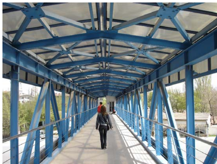
Figure 4.15 - Details of Bridge6
