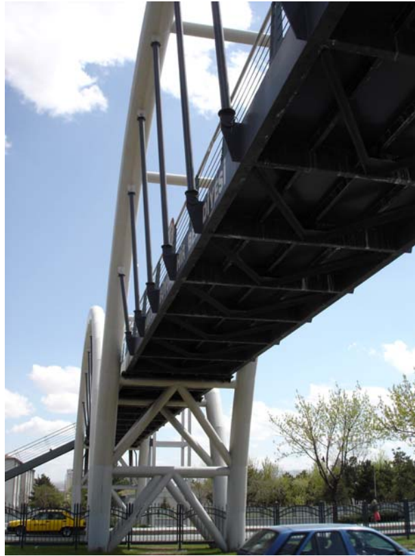
Figure 4.13 - Details of Bridge5
