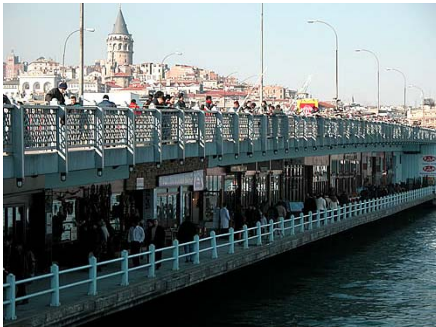
Figure 2.4 - Galata Bridge in İstanbul [19]
