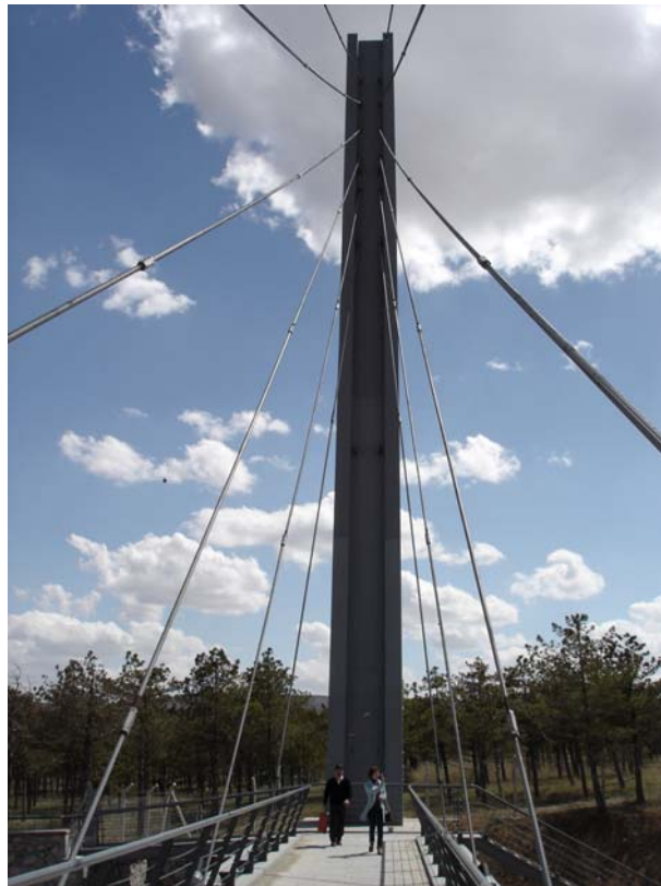
Figure 4.19 - Details of Bridge8
