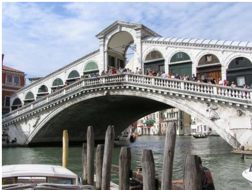
Figure 2.3 - Rialto Bridge used as an inhabited bridge, 1591 [38]
