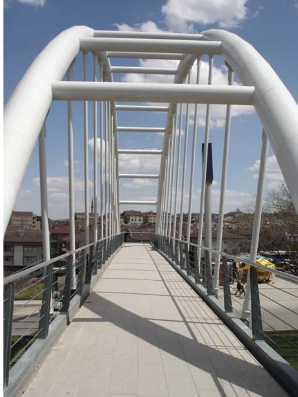
Figure 4.17 - Details of Bridge7
