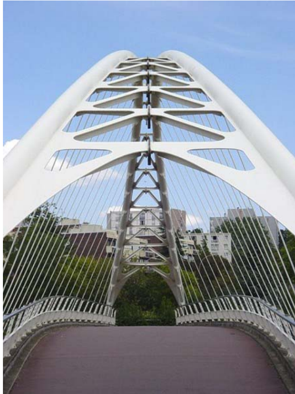
Figure 3.3 - Oudry Mesly Bridge, 1988 [38]
