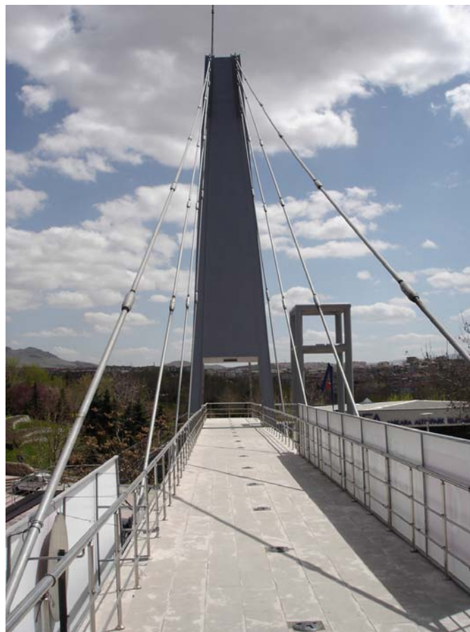
Figure 4.11 - Details of Bridge4
