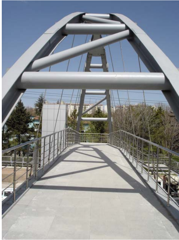
Figure 4.7 - Details of Bridge2
