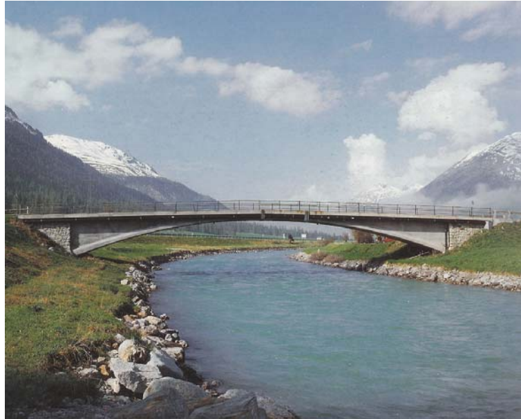
Figure 2.10 - Inn River Bridge, Zuoz [2]
