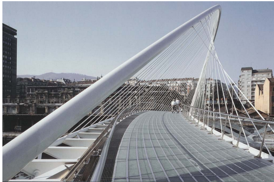
Figure 2.17 - Campo Volantin Footbridge in Bilbao, 1997 [41]
