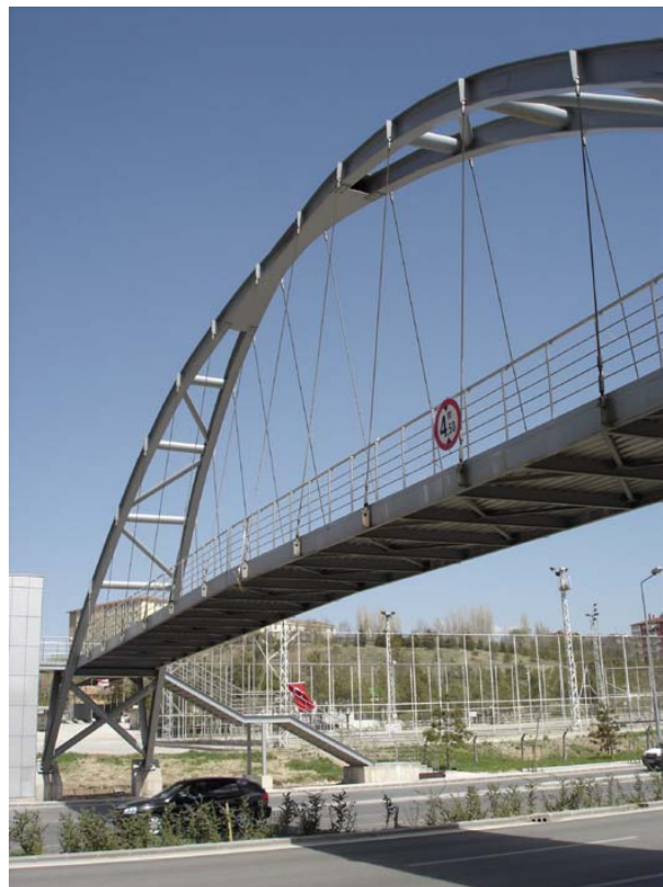
Figure 4.5 - Details of Bridge1
