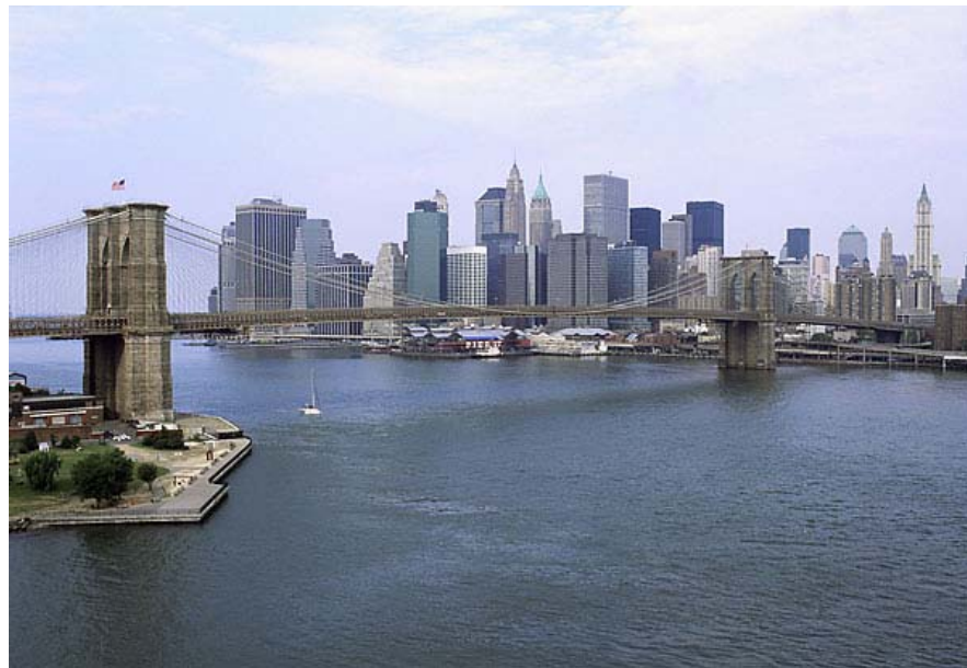
Figure 2.1 - Brooklyn Bridge in New York, 1883 [17]
