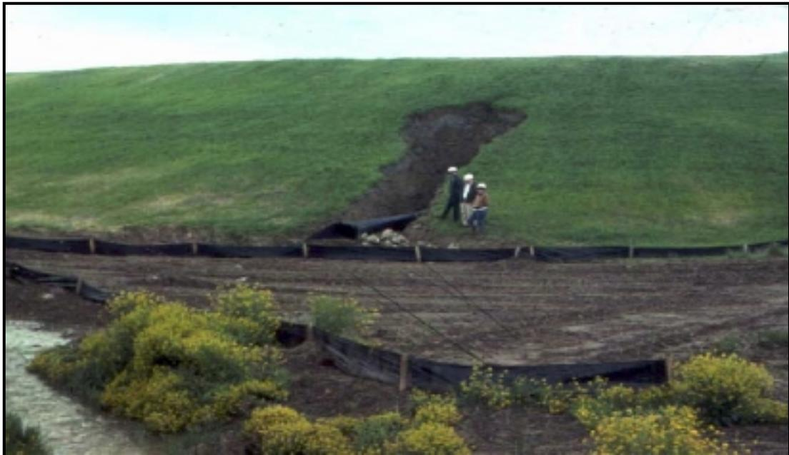
**Figure 3.6 Medford Quarry wash pond piping failure**
