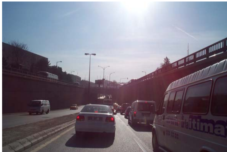
Figure 2.8 A View Taken from a Car Exiting the Akay Junction Under-pass. (Photograph by Erhan Öncü)
