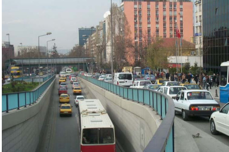
Figure 4.5 Vehicle Conflict (Photograph by Erhan Öncü)
