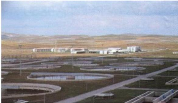
**Figure 8 Primary sedimentation tanks**
