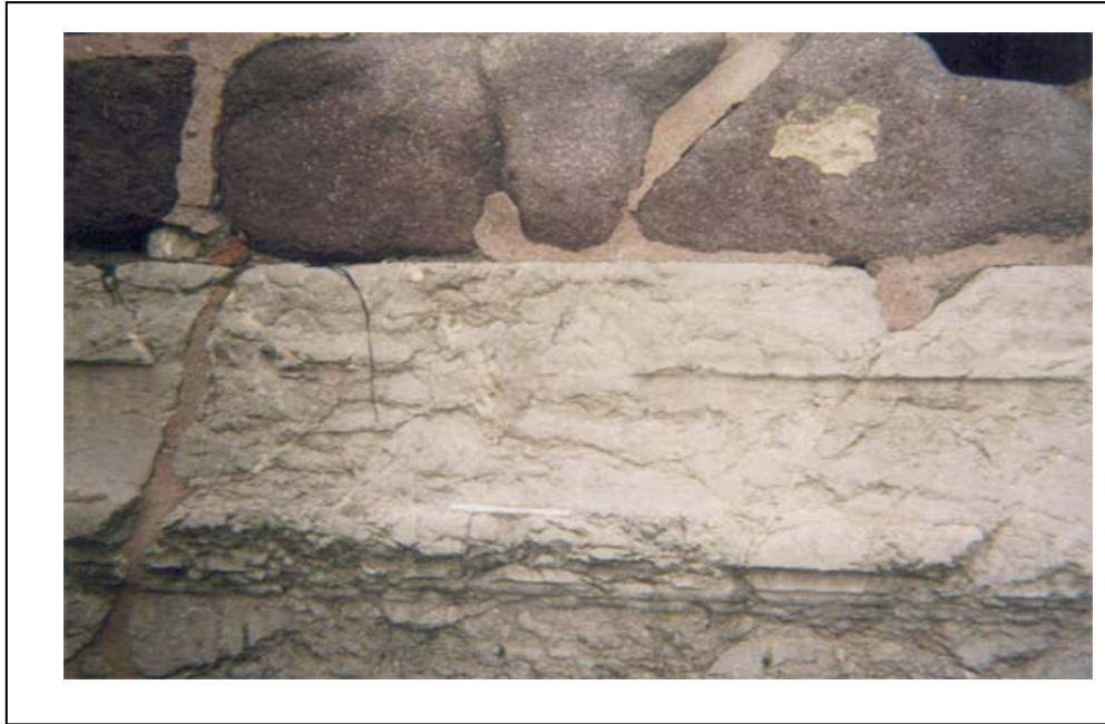
Figure 3.1 A view from west elevation at Gençkapı Gate; material loss and detachment as scales on marble surfaces
