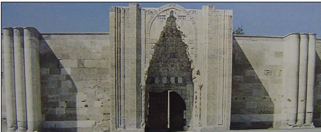
Figure 93 Sultan Han Between Konya Aksaray- Clustered Columns as Buttresses (Kuban 1999, 243)
