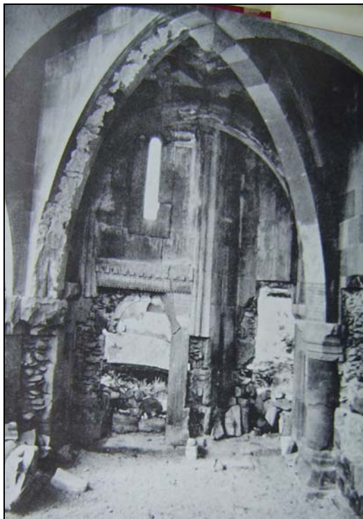
Figure 56 Church of the Apostles at Ani- Intersecting Cross Arches of the Porch (Khatchatrian 1972, Fig. 57)
