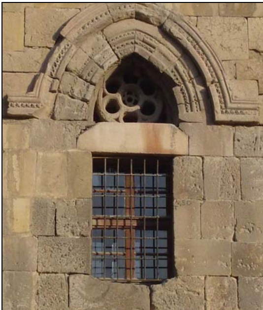
Figure 72 Sungur Bey Mosque- Recessed Arch and Tympanum of the Third Window on the South of the West Façade (D. Esin)
