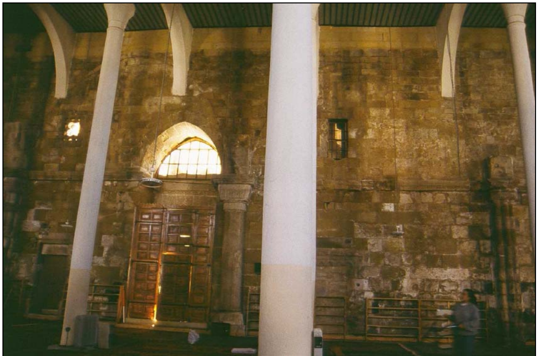
Figure 22 Sungur Bey Mosque- An Oval Column and a Cusped Pier on the East Elevation (A. Durukan Archive)
