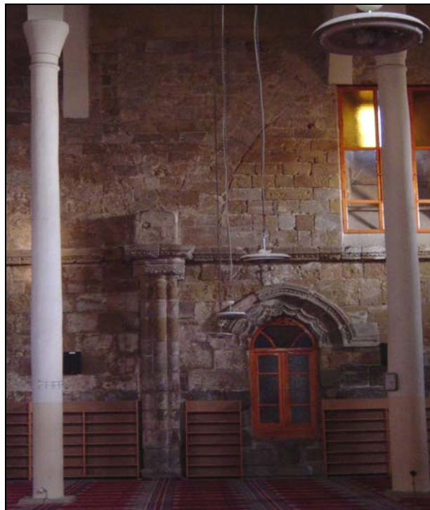
Figure 26 Sungur Bey Mosque- Window Converted to the Door of the Tomb on the East Elevation (D. Esin)
