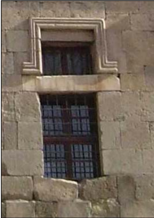
Figure 70 Sungur Bey Mosque- Recessed Arch and Tympanum of the First Window on the South of the West Façade (D. Esin)
