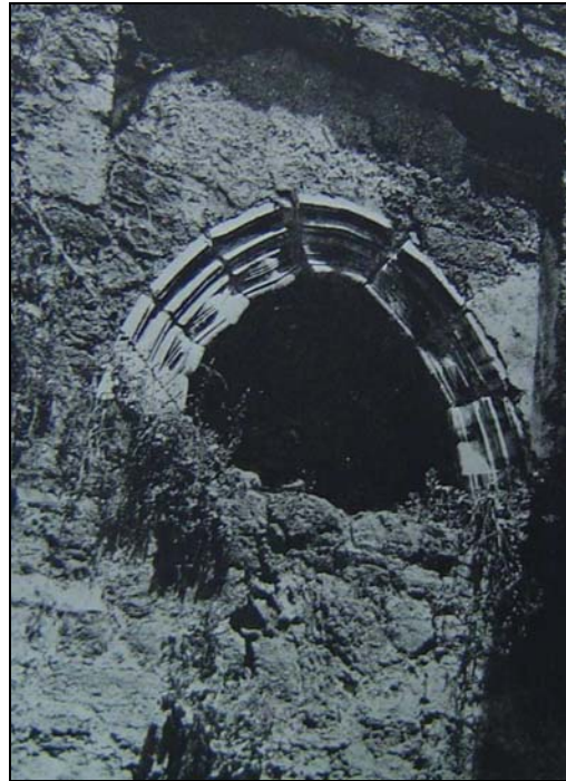
Figure 79 Ahi Yusuf Tomb in Antalya- Recessed Arch of One of the Windows (Riefstahl 1931, Fig. 91)
