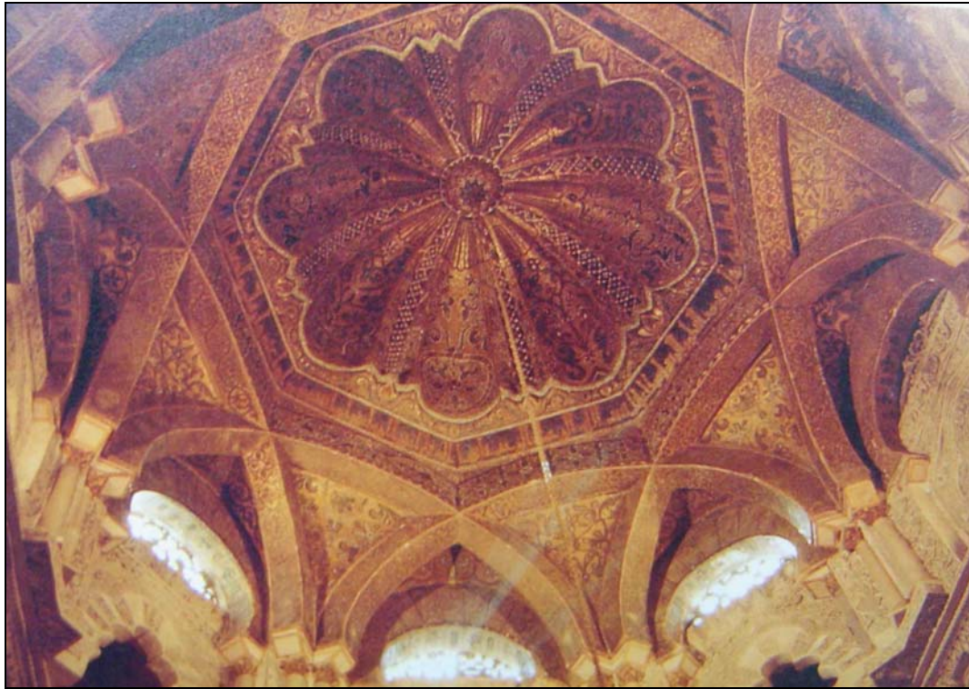
Figure 55 Great Mosque of Cordoba- Intersecting Ribs (Brend 1991, Fig. 28)
