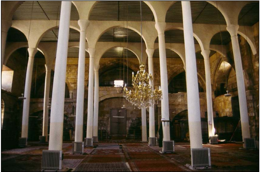
Figure 21 Sungur Bey Mosque- Timber Columns in the Interior Covered by Stucco (A. Durukan Archive)
