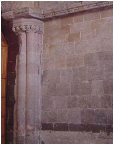
Figure 91 Sungur Bey Mosque- A Clustered Pier (D. Esin)
