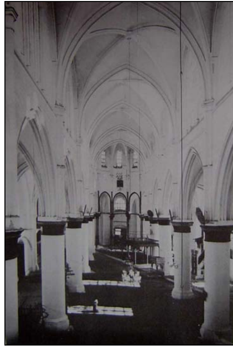
Figure 59 Cathedral of St. Sophia in Nicosia- Ribbed Vaults (Enlart 1987, Plate X)
