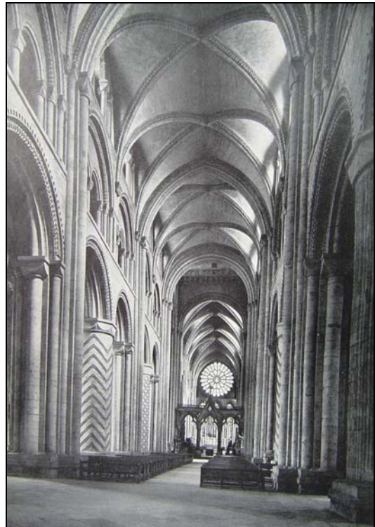
Figure 57 Durham Cathedral- Rib Vaults (Domke 1959, 4)
