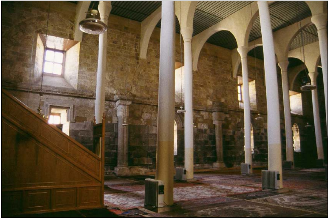
Figure 25 Sungur Bey Mosque- Windows on the West Elevation (A. Durukan Archive)
