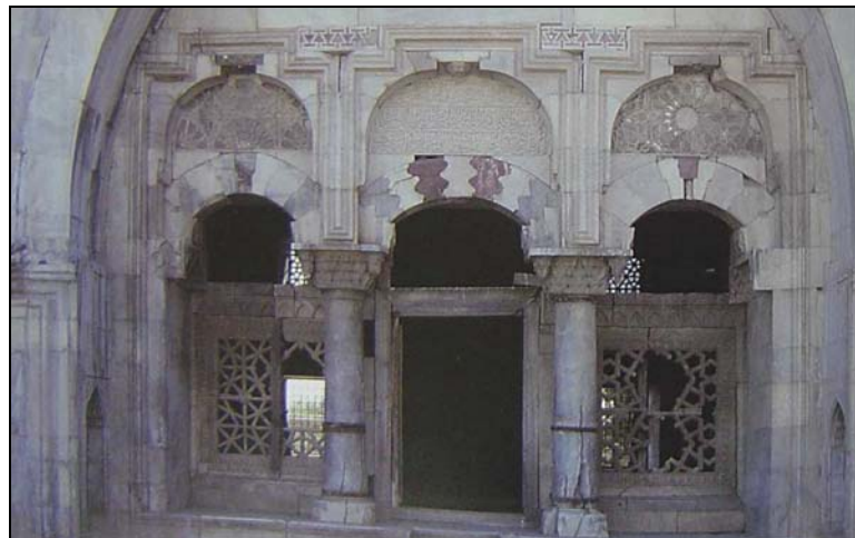
Figure 88 İlyas Bey Mosque at Balat - Marble Window Grilles at North Façade (Durukan 1988, 32 Fig. 9)
