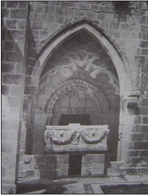
Figure 76 Bellapais Abbey in Cyprus- Recessed Arch at the Refectory (Enlart 1987, Plate XXV)
