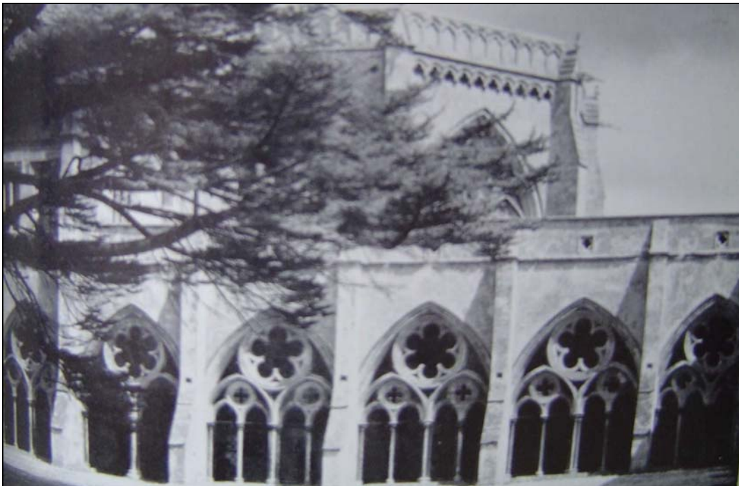
Figure 85 Salisbury Cathedral –Tracery of Arches at Cloisters (Stewart 1954,129)
