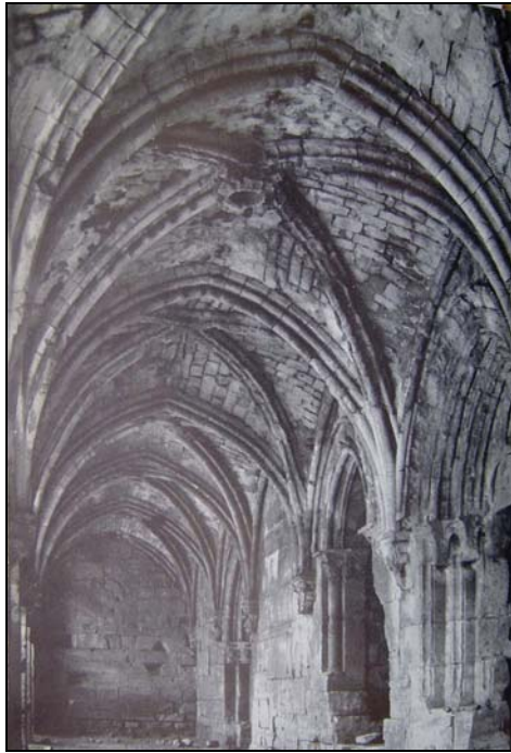
Figure 58 Castle of Krak des Chevaliers- Loggia Outside Banqueting Hall (Fedden 1957, 73)
