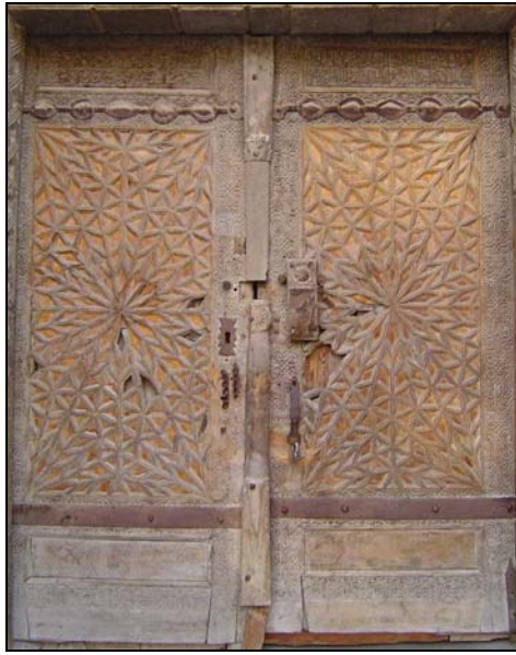
Figure 32 Sungur Bey Mosque -Wooden Door of the East Portal (D. Esin)
