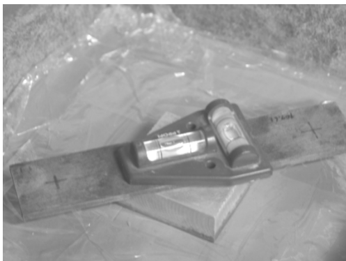
Figure 3.31 Leveling of Footing
