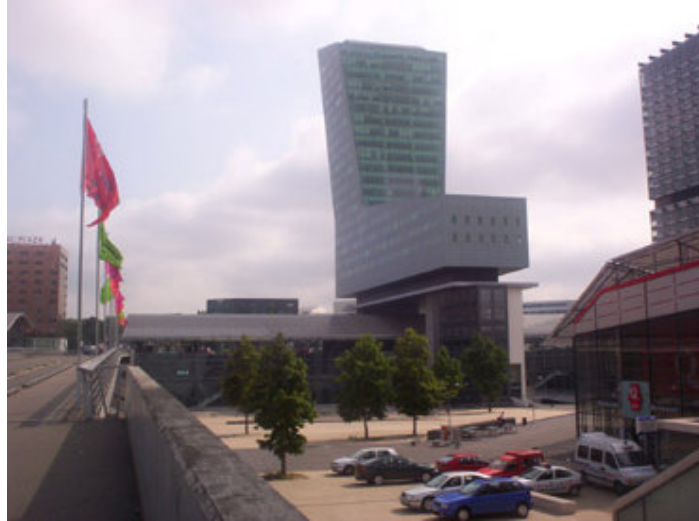
Figure 3.5.5 Lille Europe Station (Jean-Marie Duthilleul) and Credit Lyonnais Tower (Christian de Portzamparc), Euralille, 1995.
