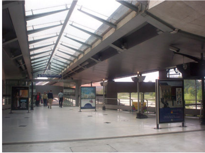
Figure 3.5.7 Connection with highway, Lille Europe Station, Euralille, 1995.
