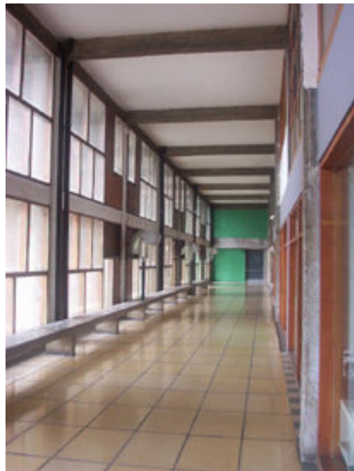
Figures 4.5.12, 4.5.13 The elevated streets (residential and commercial) set in the human scale, Unité d'Habitation in Marseille.
