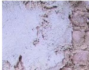
FLAKING OF PLASTER, LOSS OF FINE PLASTER
