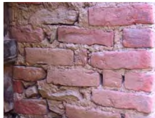
DISINTEGRATION, LOSS OF JOINTING MORTAR
