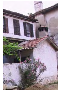
7 - Roof type 3 with French tiles is used.
