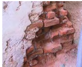
EROSION OF BRICK
