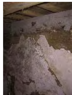
2 - Trace of altered staircase on south wall of G01 space of Çarboğa House
