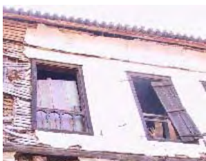
6 - Trace of removed sub elements of windows
