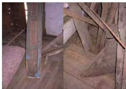
7 - Dismantled pieces of the service wall and central ceiling decoration of F02 space of Çarboğa House
