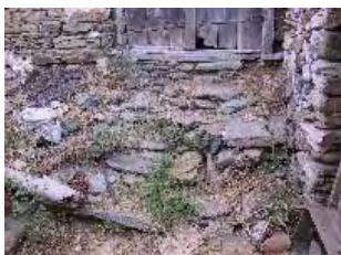
3 - Trace of removed slate stone steps
