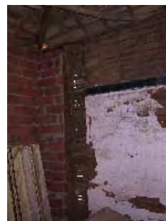
5 - Trace of removed stone masonry wall and service wall
