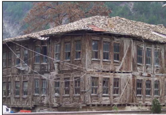
Bağdadi Construction System (Modified From Bayülke, 1934)
