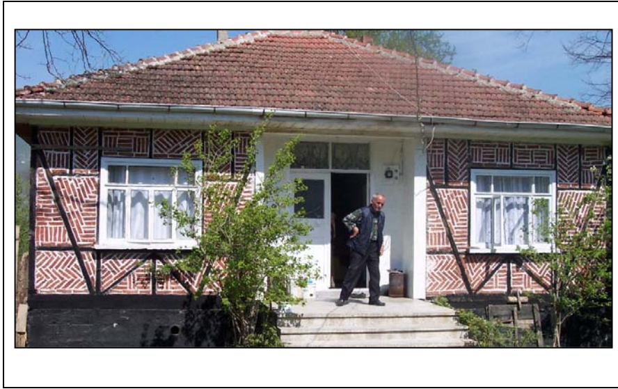
Figure 3.16 An Example of Hımış Structure with Brick Infill from Düzce
