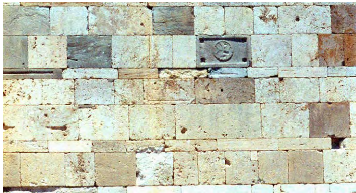
Fig. 4.2. Processed re-used face stones at south elevation
