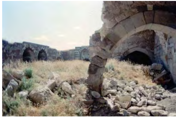
Fig. 4.46. Transition arch at Semi-open Space #3
