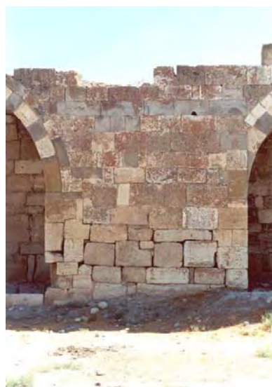
Fig. 3.24. Difference of workmanship on the south elevation of courtyard
