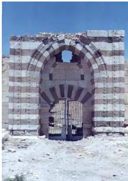
Fig. 3.14. Portal on the South Elevation (Entrance portal)
