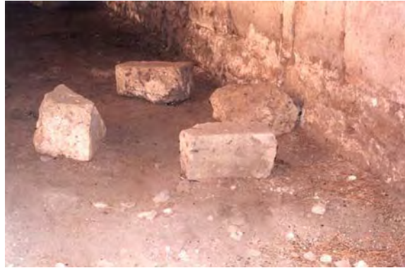
Fig. 4.32. Fallen pieces at the northeast of the Shelter
