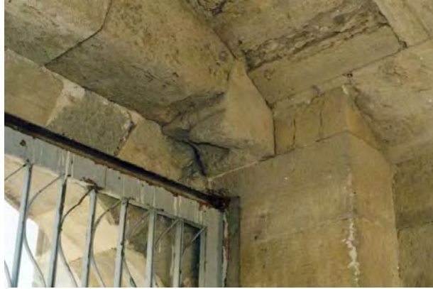
Fig. 3.29. Hinges of the Entrance door
