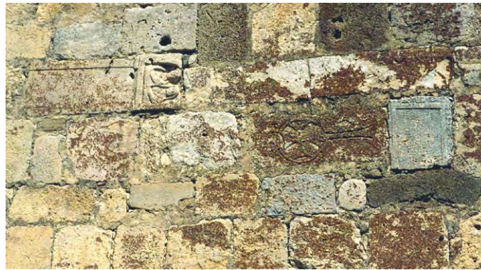
Fig. 4.3. Semi-processed re-used face stones at west elevation
