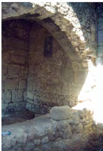
Fig. 3.34. Arched opening between Space #8 and Space #9
