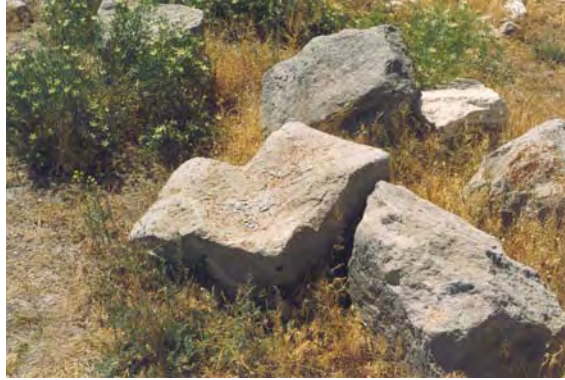
Fig. 4.35. Fallen pieces from the star vault of the Masjid
