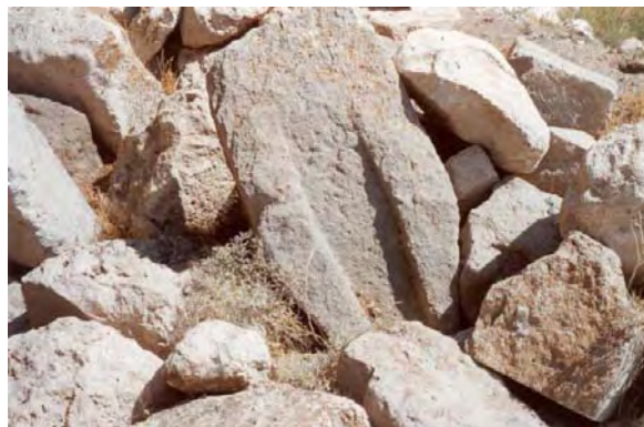
Fig. 3.41. Fallen gutter at Semi-open space #3
