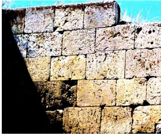
Fig. 4.1. Masons marks on the scratch built stones
