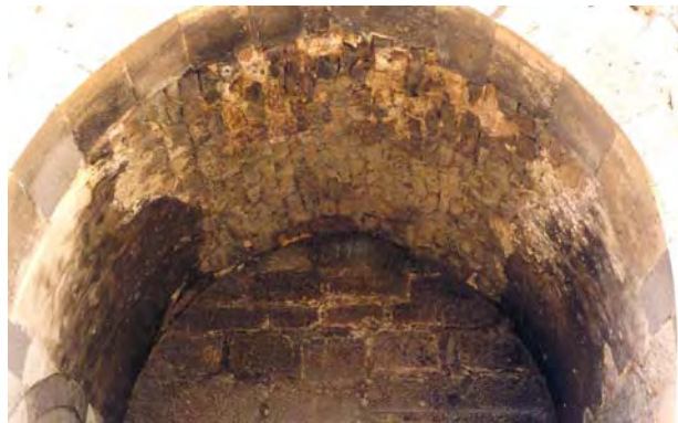
Fig. 4.9 Lime plaster at the vaults of Semi-open space #4
