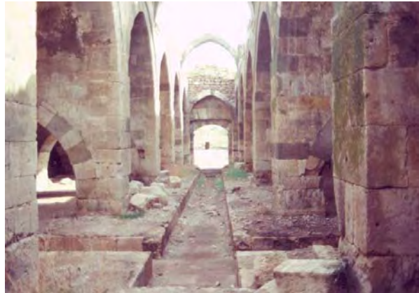
Fig. 3.47. Passage in the Shelter
