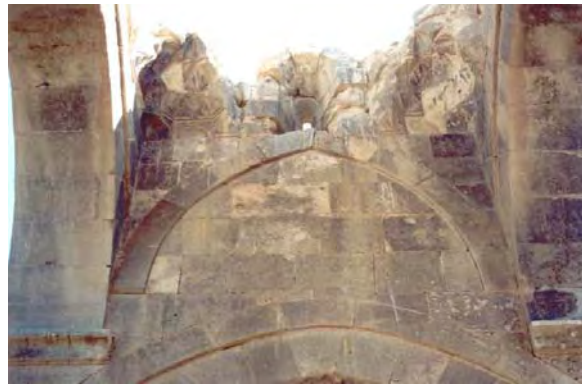
Fig. 3.45. Relieving arch on the south wall of the dome
