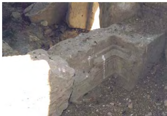
Fig. 4.34. One of the fallen cornerstones of the cornice currently locating at Space #13
