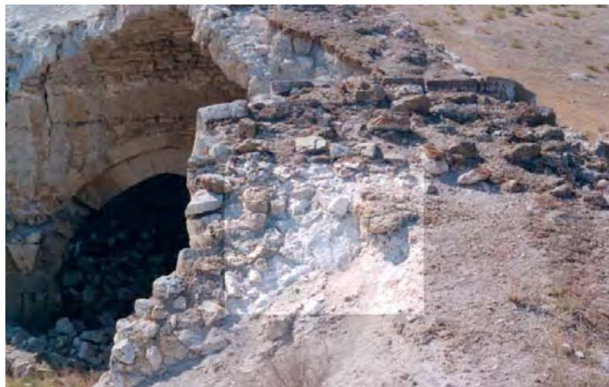
Fig. 3.49. Mortar remains at the roof of Semi-open space #3
