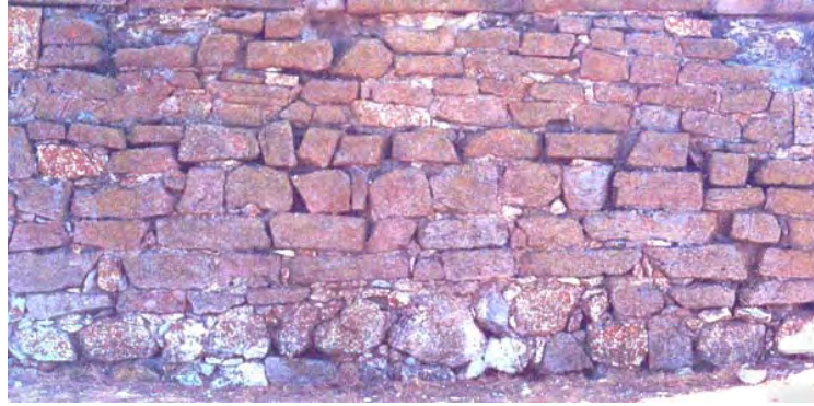
Fig. 4.5 Rough cut face stones at the north elevation of the dome
