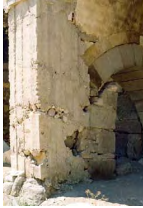
Fig. 3.42. Concrete repair at Semi-open space #4
