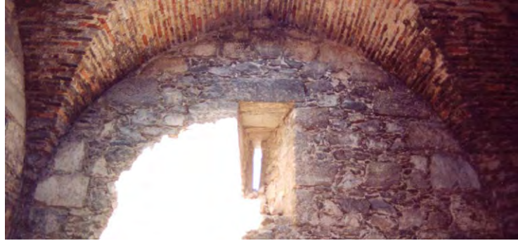
Fig. 4.8 Brick construction superstructure of Space #4
