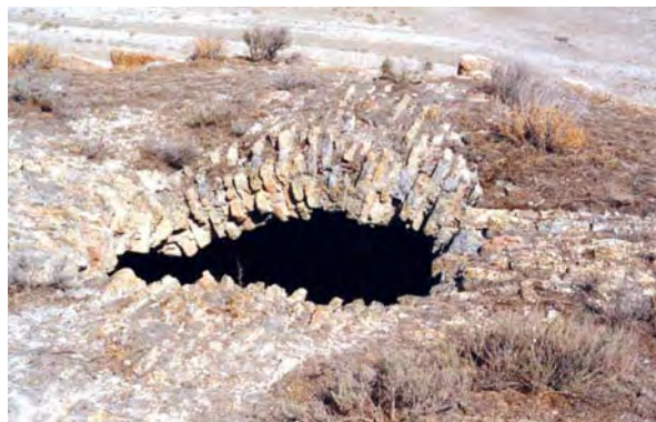
Fig. 4.28. Demolished top part of the brick construction cross vault
