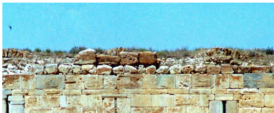
Fig. 4.4. Non-processed re-used stones on east elevation.
