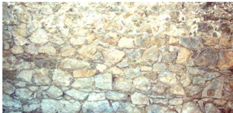
Fig. 4.6 Rubble stone wall at Space #5 interior
