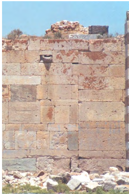
Fig.3.13. Construction joint on the South Elevation
