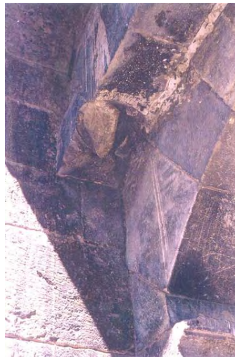
Fig. 3.46. One of the hinges of the door of the Shelter
