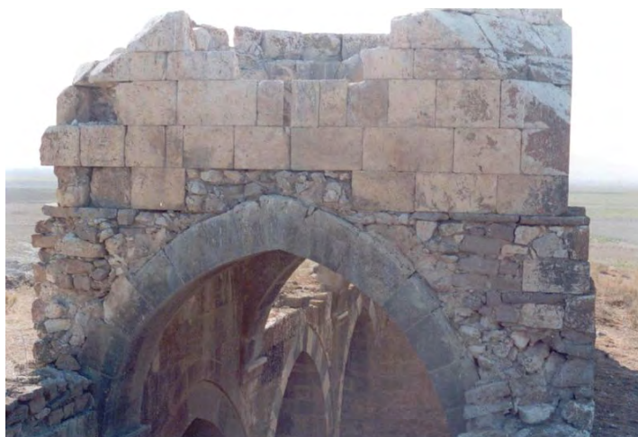
Fig. 3.50. East elevation of the dome
