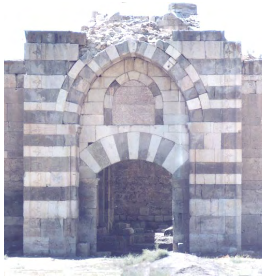
Fig. 3.27. Portal of the Shelter
