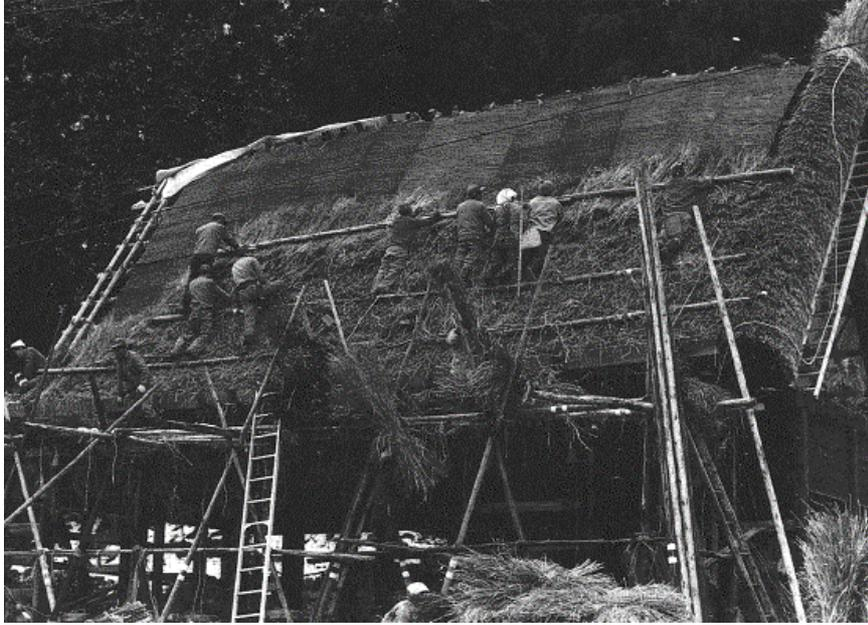
Figure 4-41 The roofing of Gassyo-zukuri
