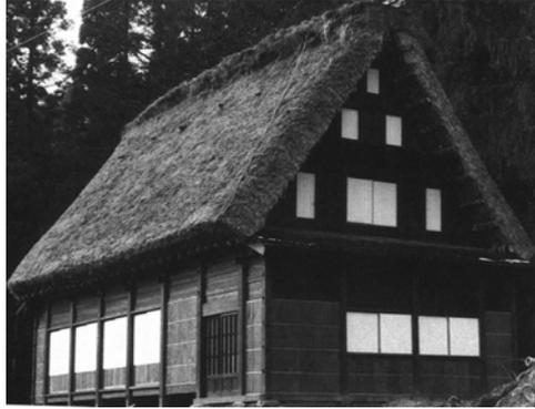
Figure 4-34 Typical exterior wall cladding of the houses in Gokayama
