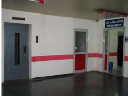
II.30.A. Entrance hall, Traffic and Traumatology Hospital, Ankara.
