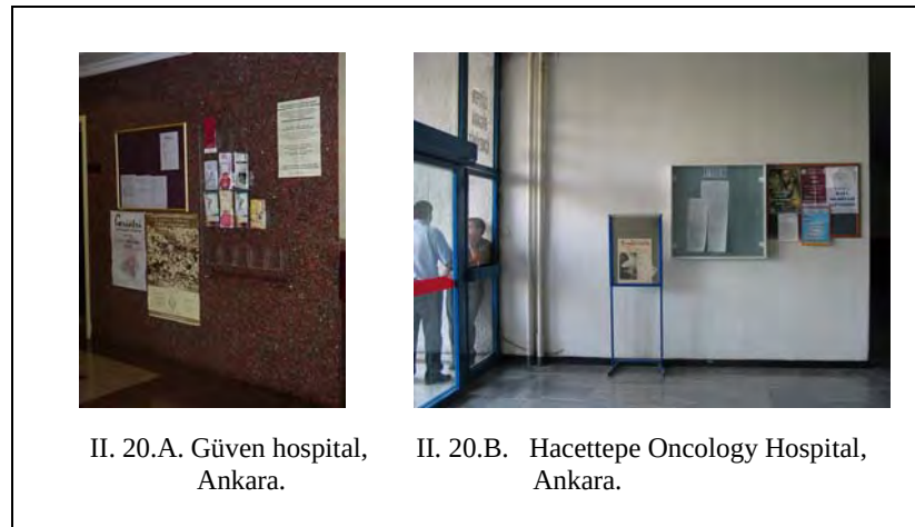
Figure II.20. Improper notice board arrangement within entrance space.
