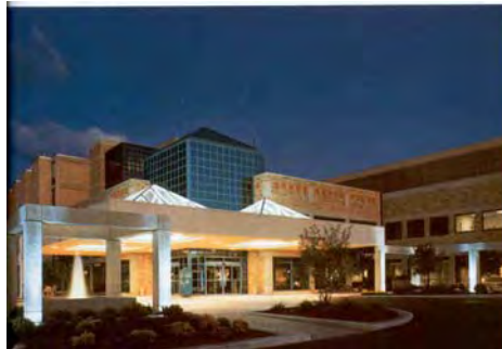
II.9.A. Memorial Hospital Addition, Seymour, Indiana (AIA, 1996: 110).
