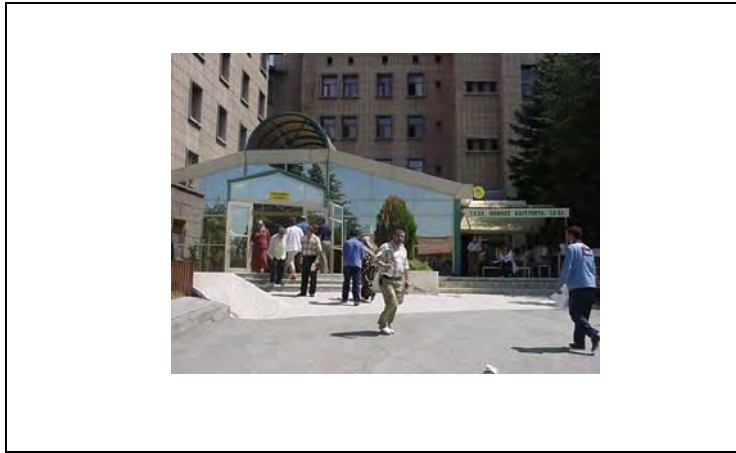
Figure II.6. An additional unit was constructed because of improper functional programming to Ankara Educational Hospital, Ankara.
