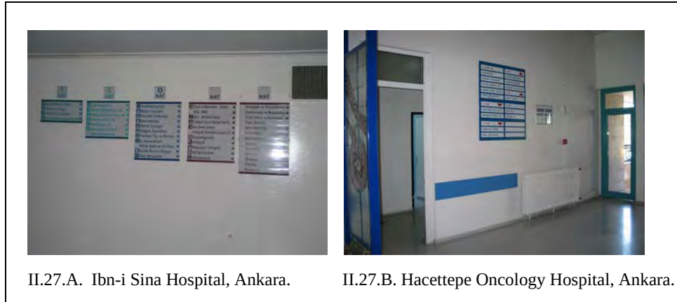
Figure II.27. Signage panels that are not designed and organized properly.
