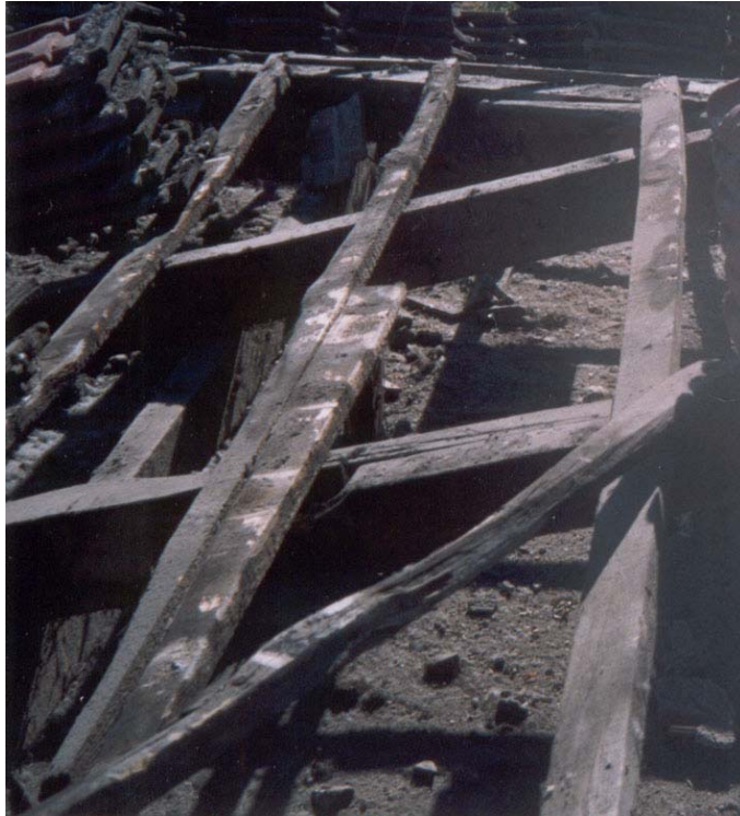
Figure 4.7 Defects on timber components occurred during its first usage.
