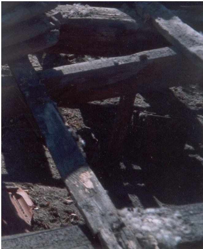
Figure 4.8 Defects on timber components occurred during its first usage.
