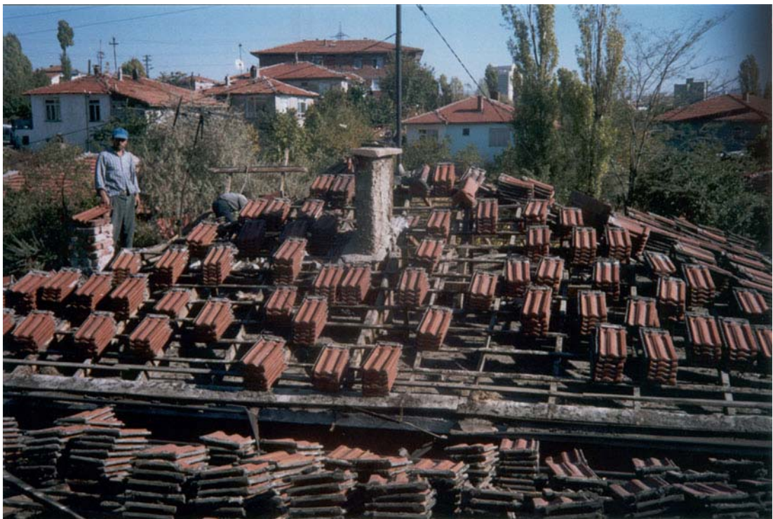
Figure 4.11 Selective dismantling of roofing tiles on the roof.
