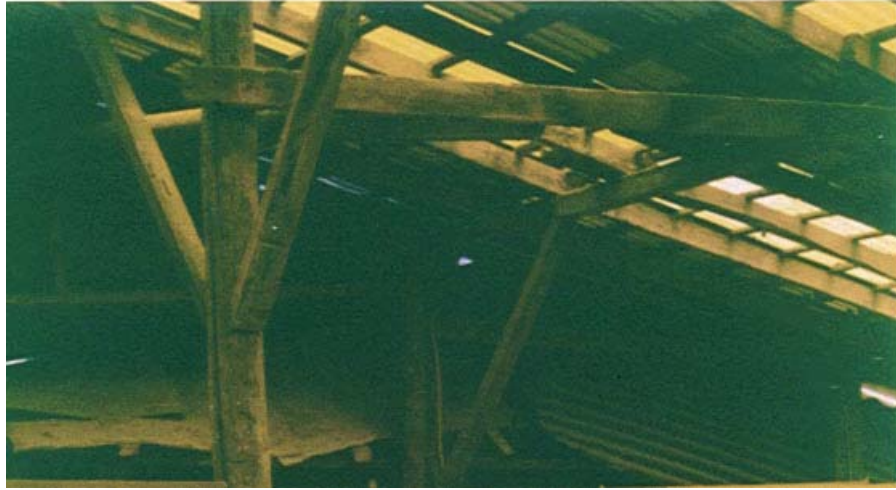
Figure 4.6 Re-use of reclaimed timber in the display area of contractors in Bentderesi.
