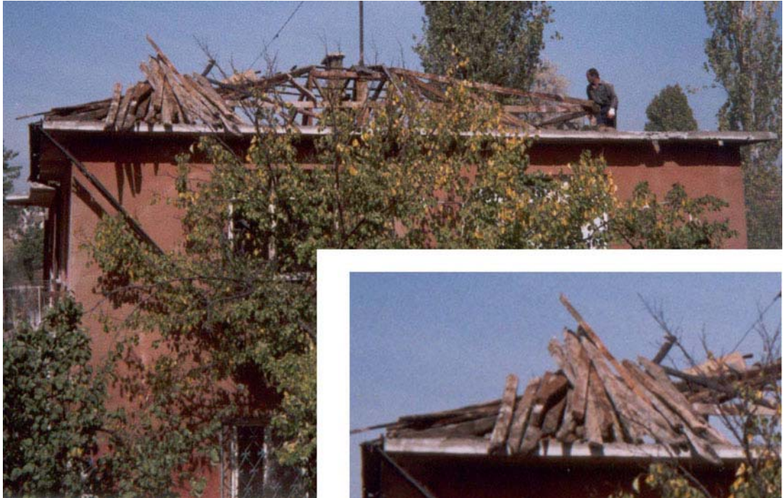
Figure 4.10 Selective dismantling of roof timber structural elements, lack of storage area on Site.
